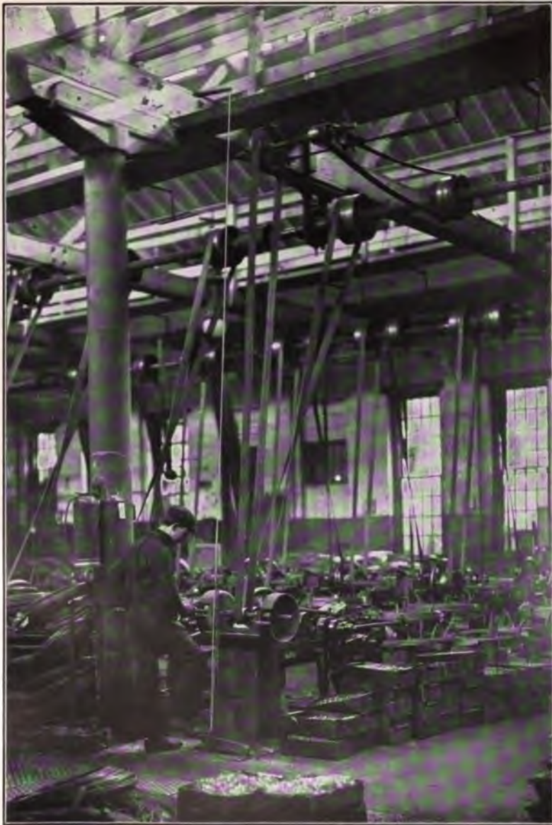
PLATE II.—VIEW IN NAIL MILL SHOWING SAFETY HOODS OVER EMERY GRINDERS, WHICH ARE FLANGED OUT OF A SOLID PIECE OF STEEL PLATE
